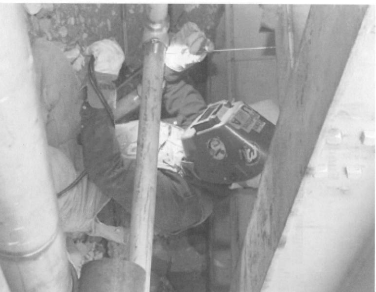
Pipefitter working in close quarters.
